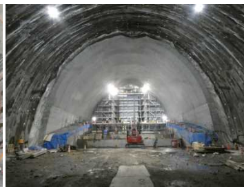
減勢池部施工状況 (H31.2)
