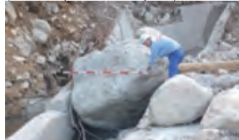
Implementation of investigation of the disaster situation of collapsed rivers (2017 Heavy rain in North Kyushu)
