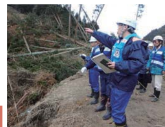
Local Government Support Activities (Technical support by TEC-FORCE, Miyazu City, Kyoto Prefecture)
