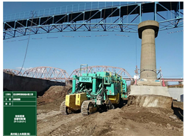
写真-2 岩盤切削機(2500SM)
