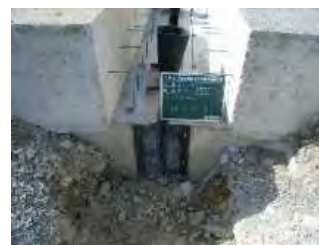
(防砂板設置状況)
