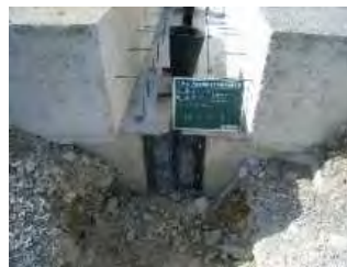
(防砂板設置状況)
